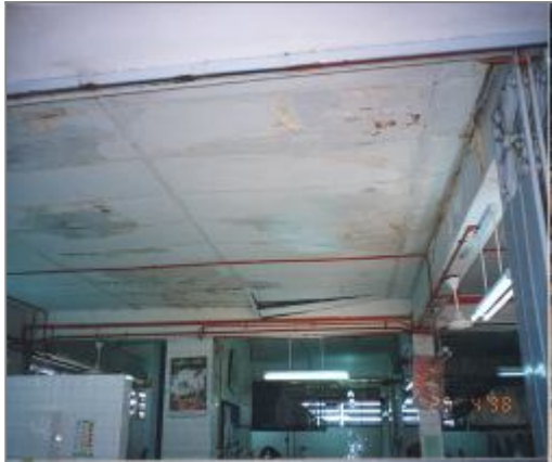
Before paint job
